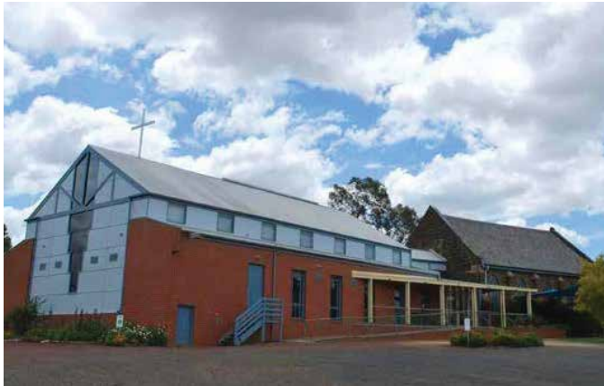
Melton Uniting Church, Melton
